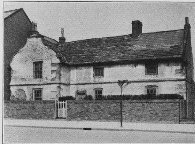
OLD COTTAGE, NEAR ST. LUKE'S CHURCH.
